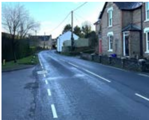
Existing view of North Street (looking south)
