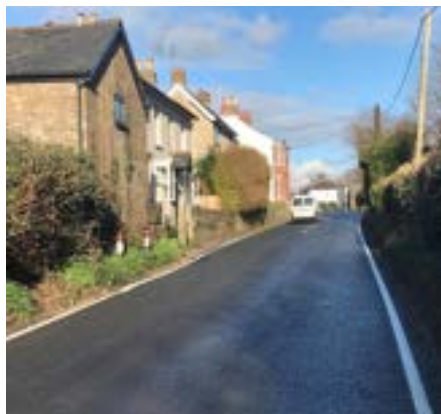
Existing view of North Street (looking north)
